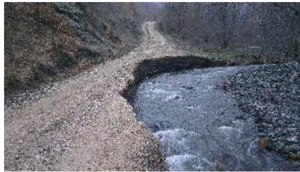
Fig.6. Typical example of a road damaged by flood (March 2013)
