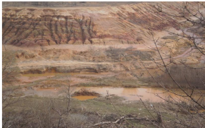
Fig.7. Industrial Waste Landfill with erosion faults on the river Ibar bank
