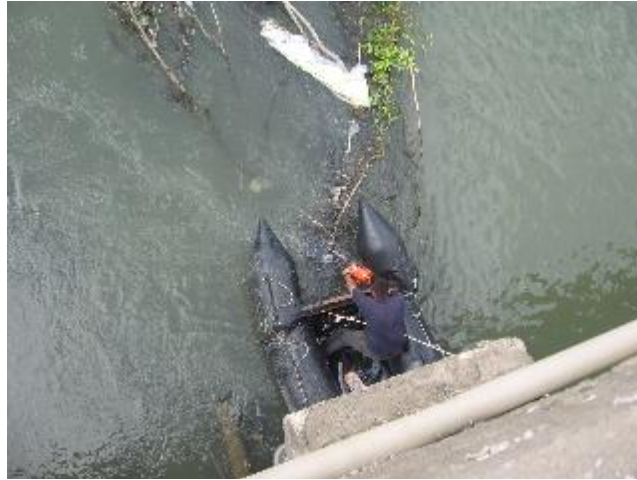
Fig. 3. Damaged Dam in Leposavic due to the floods in 2014
