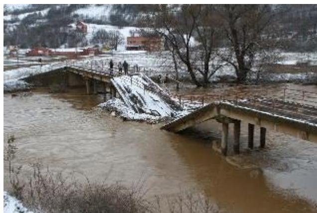
Fig.5. Broken bridge in Kutnje, 2013
